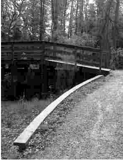
Approach to 2nd. Bridge # 24 & 23
