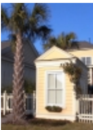
Jakes Lane Outbuilding # 4
